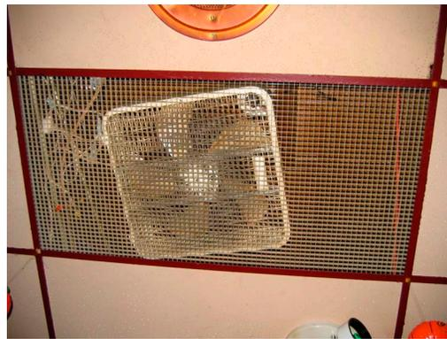
Figure 3. Fan laying on ceiling panel in bar area
